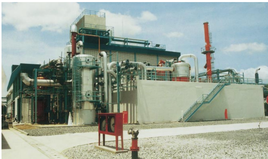
New sulfation plant for the production of surfactants in Thailand. The plant incorporates the latest technology and is environmentally compatible. It is located on Henkel Thailand's new 80,000 square meter lot.
