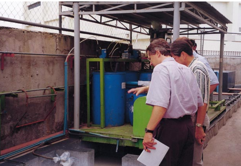
Independent auditors check the safety status and the efficiency of environmental protection at a wastewater pretreatment plant operated by Henkel Philippines.
